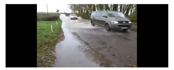
At present in times of rain, water collects at edge of the proposed site and does not flow into the channels that surround the area. The existing culvert under Church Road is inadequate for the road as it is now, and further development of the surrounding area without significant investment or change in the drainage infrastructure will result in this recurrent issue becoming more frequent.
